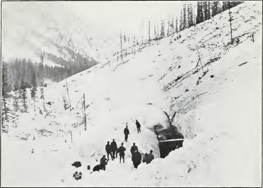
FIG. 1.—CLEARING SNOW AND DÉBRIS FROM THE RAILROAD TRACKS AFTER THE BERNE SLIDE, WHICH CAME FROM THE DEFORESTED HILLSIDE ON THE RIGHT AND COVERED THE TRACK FOR A THIRD OF A MILE.
